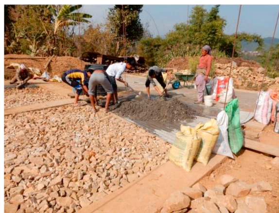
Fig. 5. Construction of the foundation and damp proofing course of a house.
