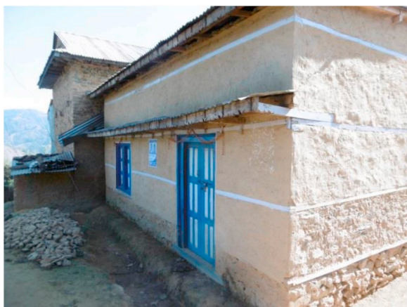
Fig. 7. Rebuilt house after the earthquake.
