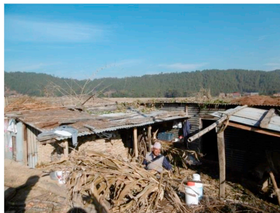
Fig. 4. Temporary houses made of CGI sheets after the earthquake.
