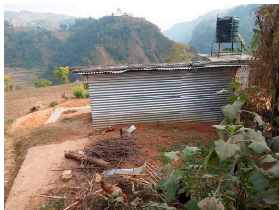
Fig. 8. Temporary house made of materials provided by the government after the earthquake.
