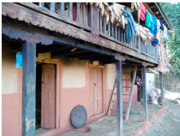
Fig. 9. Repaired house after the earthquake.
