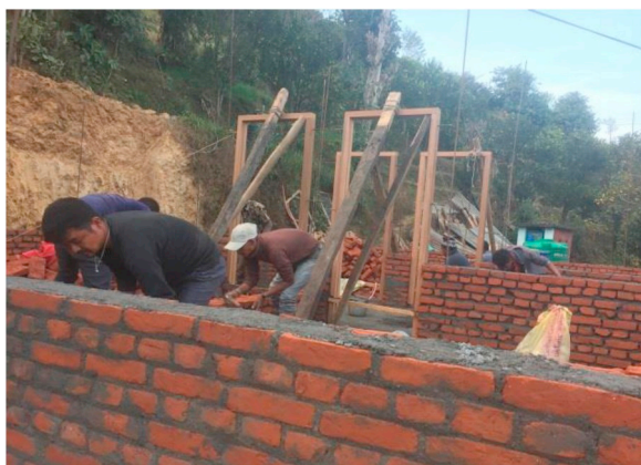
Fig. 6. Construction of the wall of a house.
