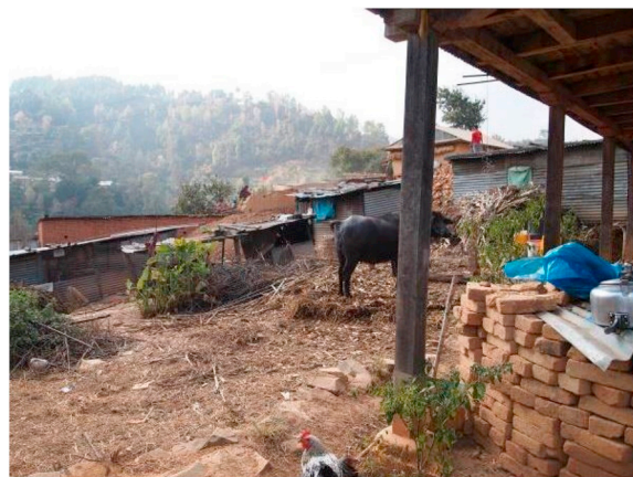
Fig. 11. Livestock raised in front of an unrepaired house.
